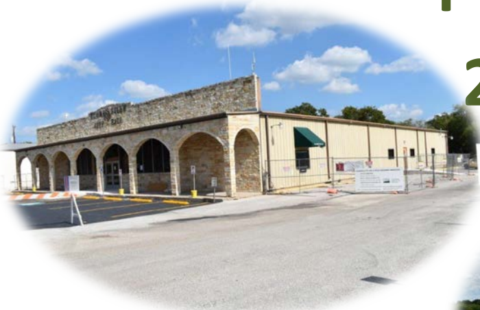
CITY HALL REPAIRS
