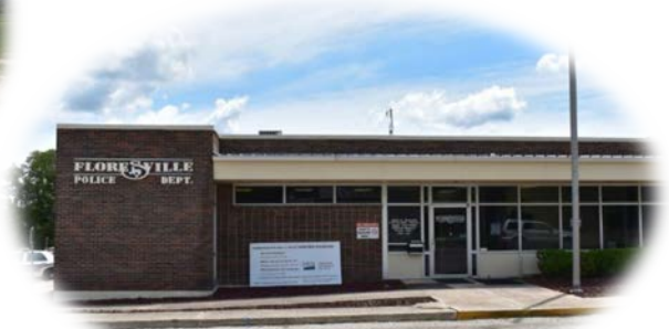
POLICE DEPARTMENT REPAIRS
