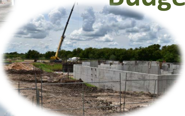
SEWER PLANT CONSTRUCTION
